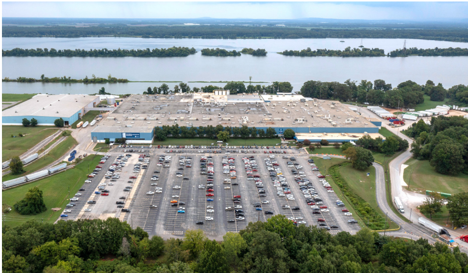
GE Appliances Refrigeration Plant in Decatur, AL.
